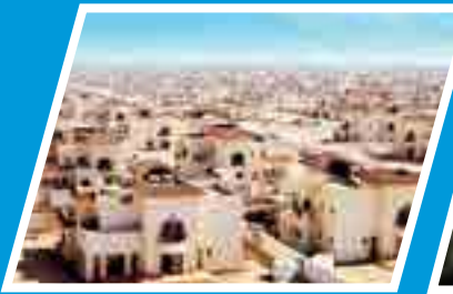
Emirati Housing Development City: Al Ain, U.A.E Total Capacity: 80,000 HP
